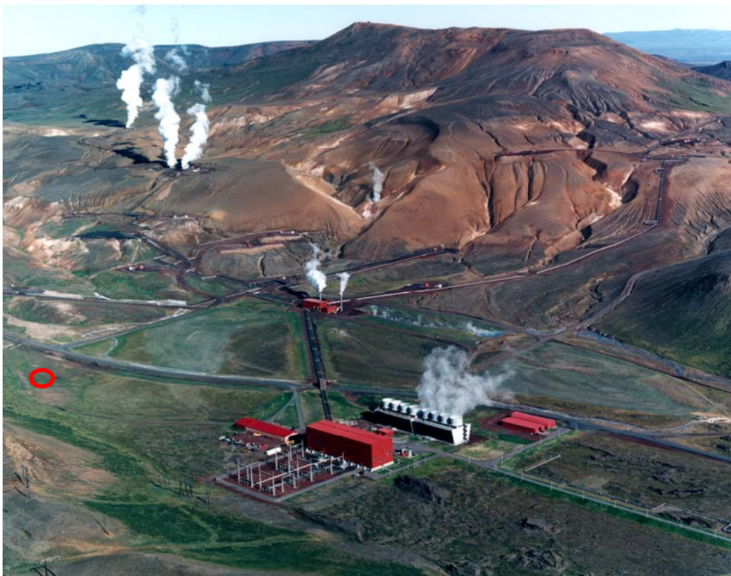
A view to the Krafla Central Volcano. A 60 MW power plant is seen in the foreground. The red circle denotes the potential IDDP drillsite.
