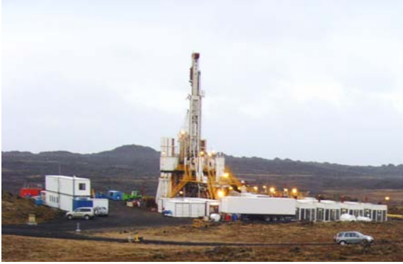
Figure 7: The Drilling Rig Tyr at Borehole RN-17.
